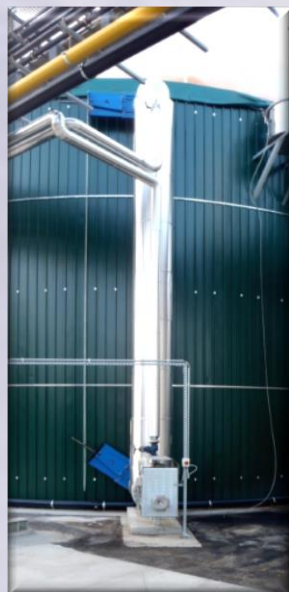
Digestmix® , a unique mixing & heating system
