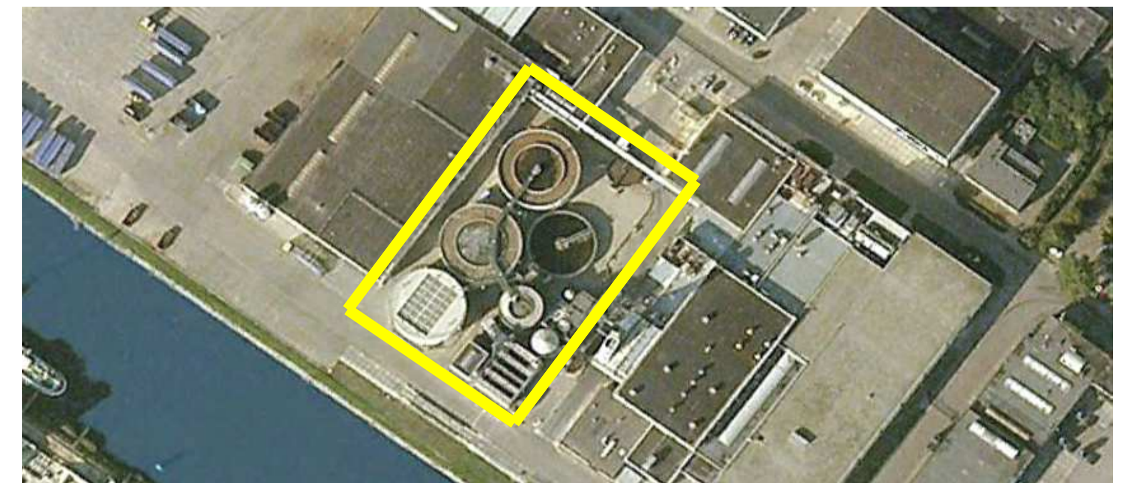
Figure 2: Aerial view of WWTP at LWM, Bergen op Zoom (The Netherlands)
