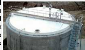
SBR-NAS reactor (Salamanca ES)
